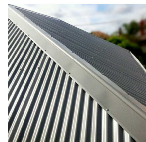
4. BLUESCOPE ZINCALUME ROOFING - SPANDEK PROFILE
