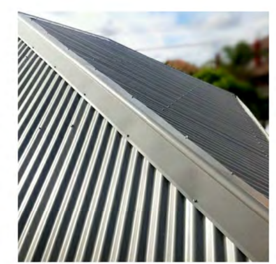
3. BLUESCOPE ZINCALUME ROOFING - SPANDEK PROFILE
